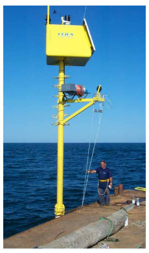
One of the service that Floatex grants to its customers is the after-sales assistance. Once a buoy is delivered, it still has to be deployed. Floatex technicians are available for assisting the correct on site installation of the delivered products. Supervision from Floatex technician have been carried out in the past for installation of mooring buoys, elastic/ articulated beacons and GRP towers, just to make some examples.
